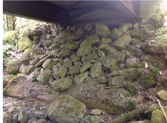
Right Bank Abutment when facing downstream
