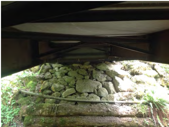
superstructure and left abutment
