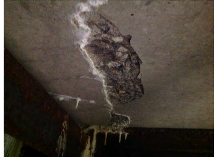
spalling concrete
